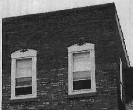
Historic ornament (the upper cornice and possibly the window hoods) has been removed. The eagles add some decoration, but are not historically accurate. The original windows have been replaced with windows that are too small for the original opening.
