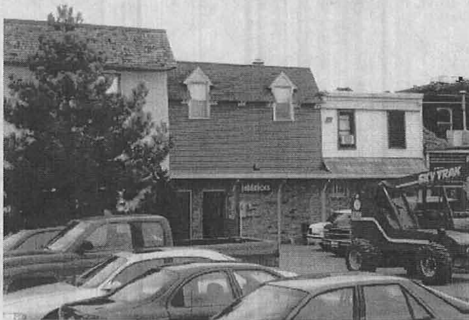
These rear facades have inappropriate residential detail and materials.
