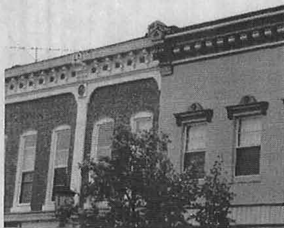
The cornice at left appears to be original. The cornice at right is a reconstruction that seems accurate on the whole. Always base reconstructed ornament on photographic evidence rather than conjecture. For instance, the semicircular elements over the window hoods on the right are questionable.
