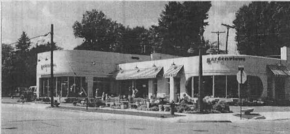
A sensitive re-use for this modern building. The awnings are not historically accurate details but the remainder has been kept largely intact.
