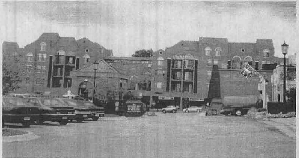
This large building has been divided into smaller masses. The overall effect of the building is still very massive because of the scale, height, and homogeneity of materials in relationship to the neighboring buildings.
