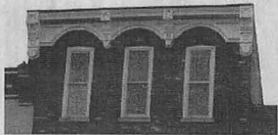
A well preserved upper cornice is a major character defining feature.
